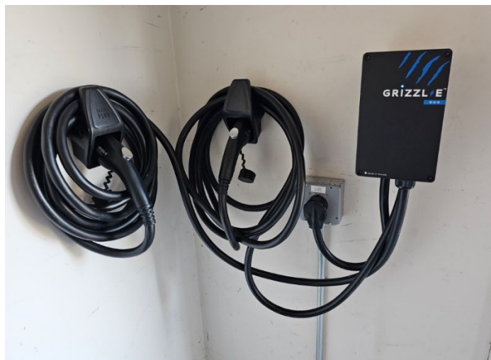
A home charging setup for two EVs from a single NEMA 14-50 outlet offers power sharing for optimal load management as more homes adopt a second and third EV
