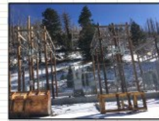
San Antonio: Large amount of fire fuel (timber and debris) piled up near the equipment.
