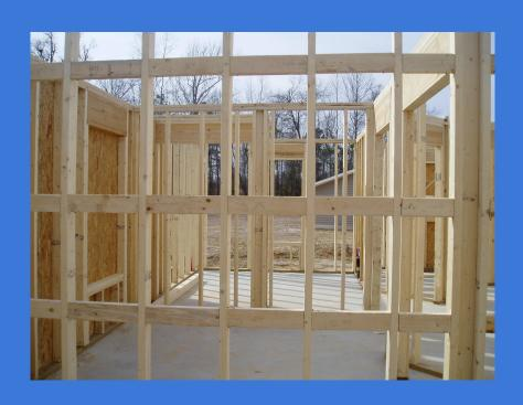
Wall framing is the process of attaching building materials together to create a structure like a wall.
