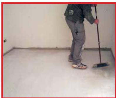
5. All sub-floors should be tested for relative humidity with an accurate testing apparatus. The relative humidity of the sub-floor should be no greater than 75% (as per ASTM F2170). If the sub-floor is above the acceptable limits, a suitable moisture barrier system should be applied to the sub-floor and allowed to cure, prior to the application of this adhesive.
