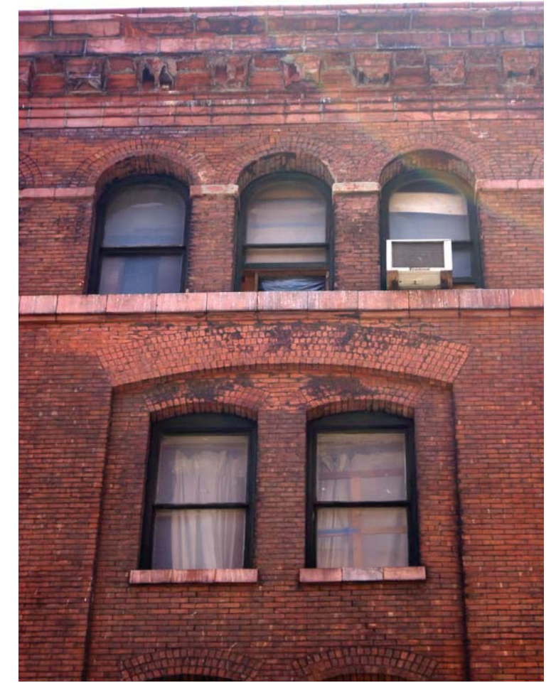
401 WASHINGTON STREET, DETAIL BRICKWORK AND CORNICE
