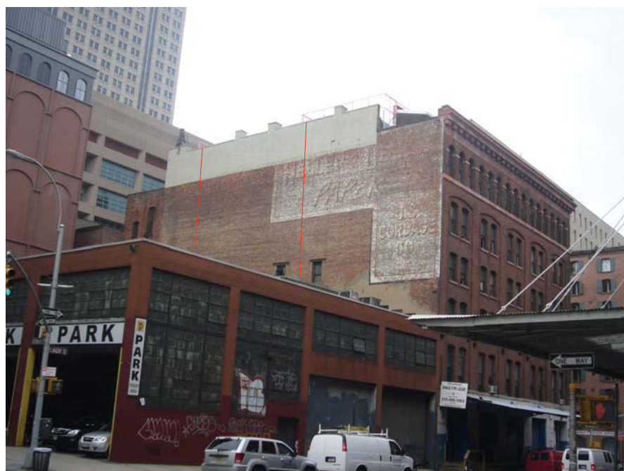
3, VIEW FROM GREENWICH & LAIGHT STREET
