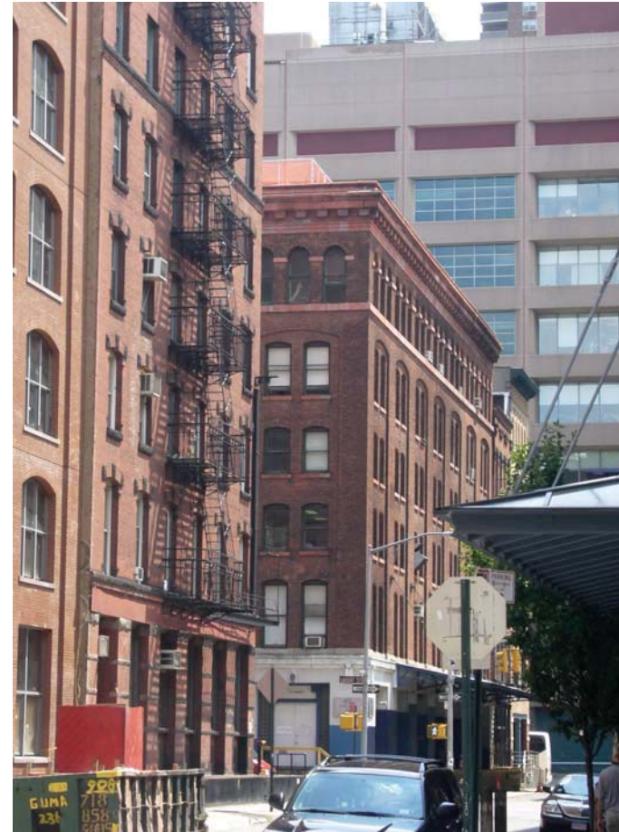
2, VIEW FROM WASHINGTON STREET
