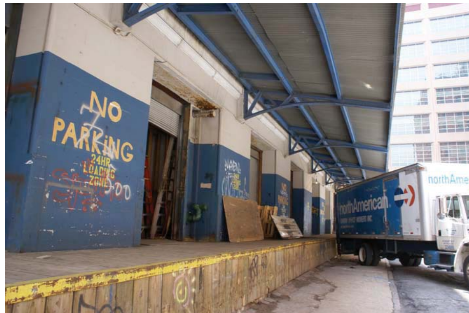
401 WASHINGTON STREET, LOADING DOCK ON WASHINGTON STREET
