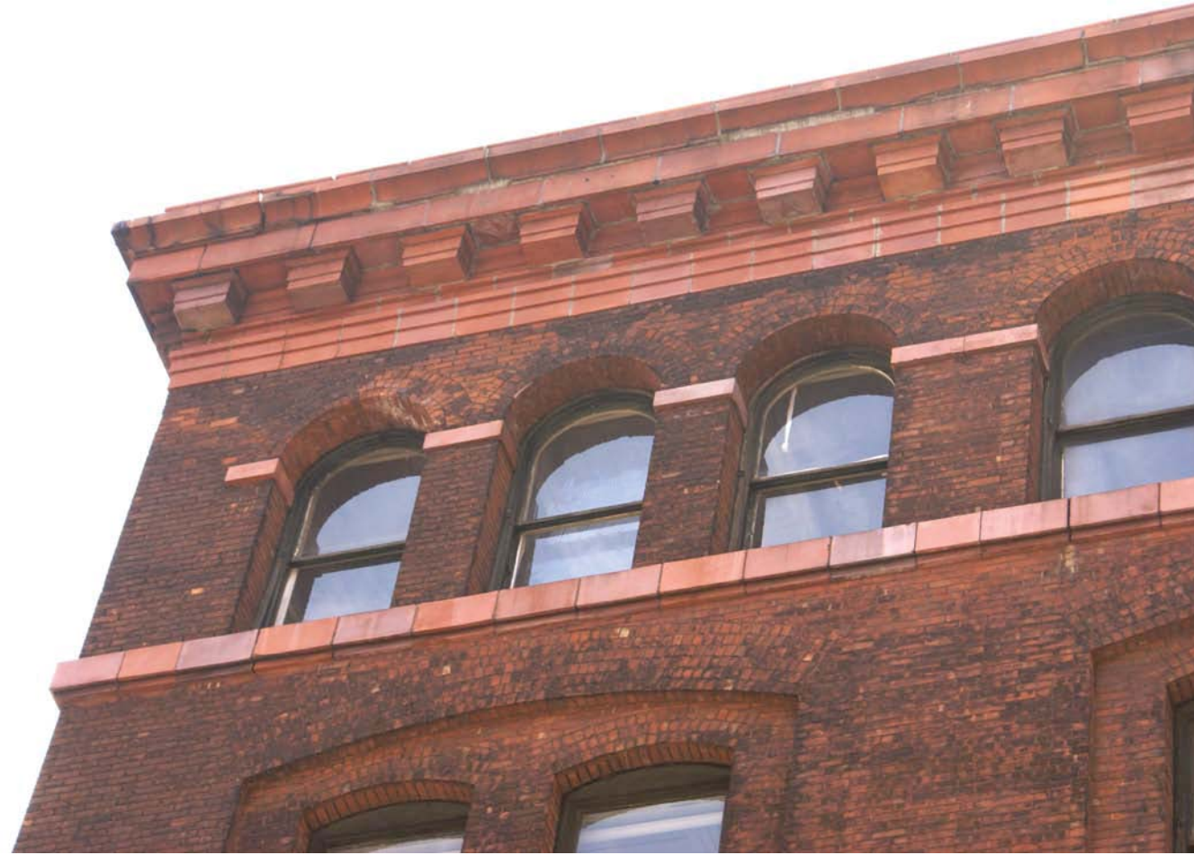
401 WASHINGTON STREET, DETAIL BRICKWORK AND CORNICE
