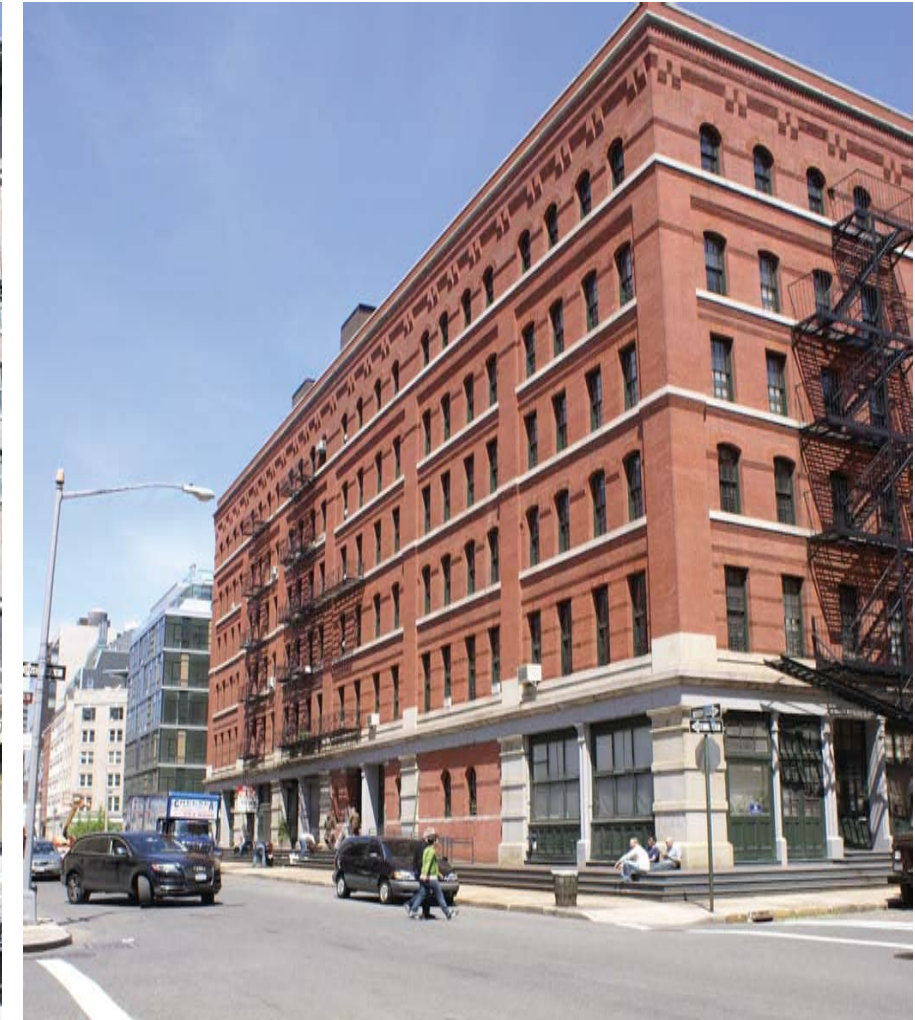
③ 461-469 GREENWICH ST / 18-22 DESBROSSES ST / 125-129 WATTS STREET, 1884-1885
