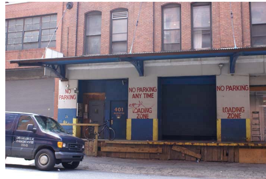
401 WASHINGTON STREET, LOADING DOCK ON LAIGHT STREET
