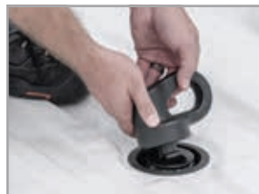
Step 3 - Drop in each anchor and twist 1/4-turn
