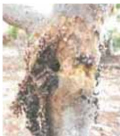
Excreta with web around bored hole
