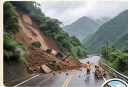
Landslides & Critical Infrastructure Failure
