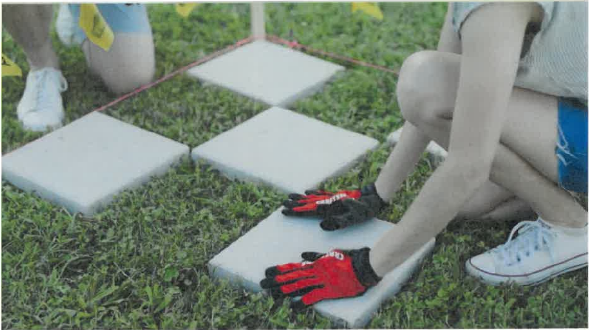
Fig. 3 – Example of layout and installation of checkerboard
