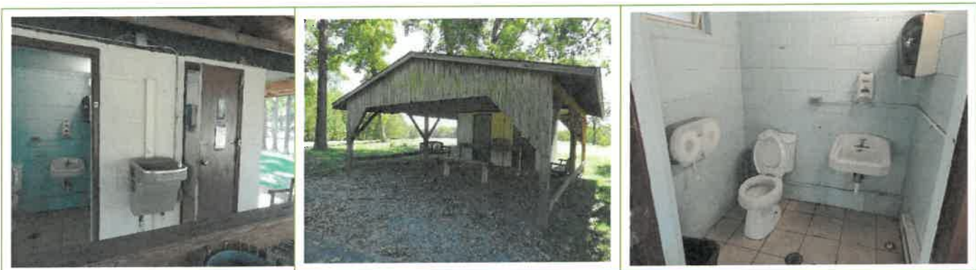
Images of on-course services at JPGC showing extremely poor conditions. Restrooms and drinking stations are being replaced in 2022.
