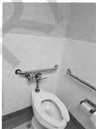
Figure 31: Jamestown Fire Station Toilet Room Grab Bar View 2
