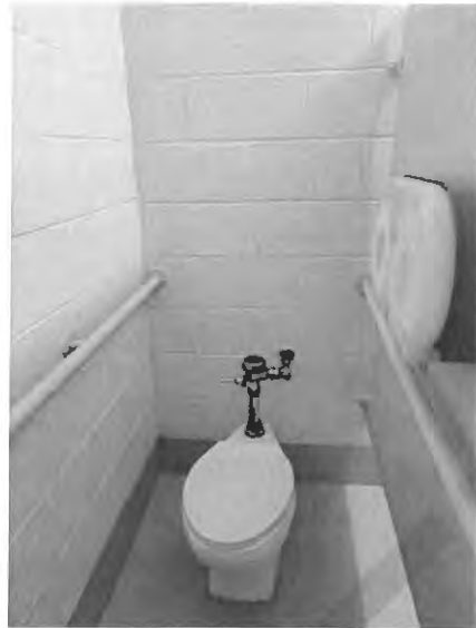
Figure 64: Jamestown Public Park Toilet Room Stall View 1
