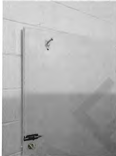
Figure 61: Jamestown Public Park Women's Bathroom Coat Hook
