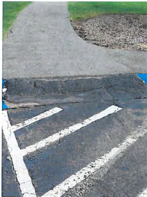
Figure 47: Jamestown Public Park Access Ramp View 2
