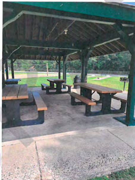
Figure 54: Jamestown Public Park Seating Area View 2
