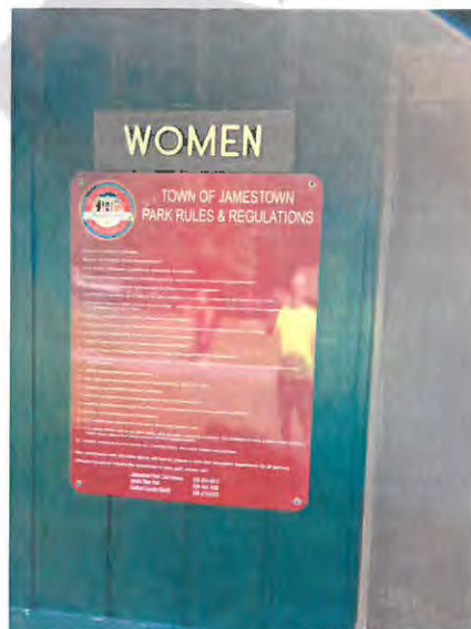
Figure 56: Jamestown Public Park Women's Toilet Room Sign
