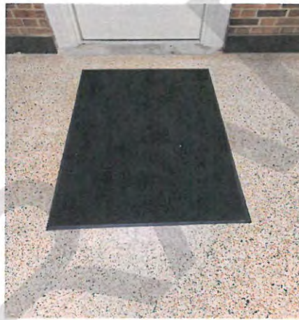
Figure 83: Jamestown Town Hall Entrance Mat 1
