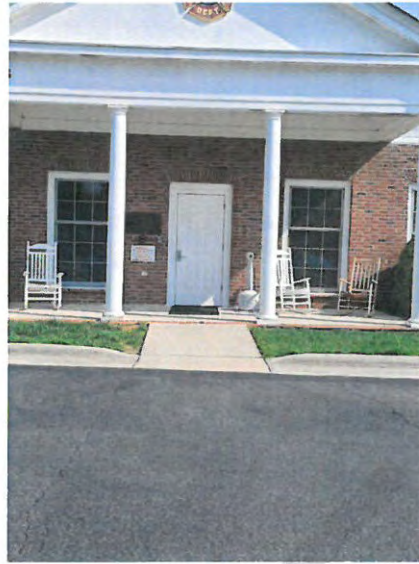
Figure 20: Jamestown Fire Station Accessible Entrance
