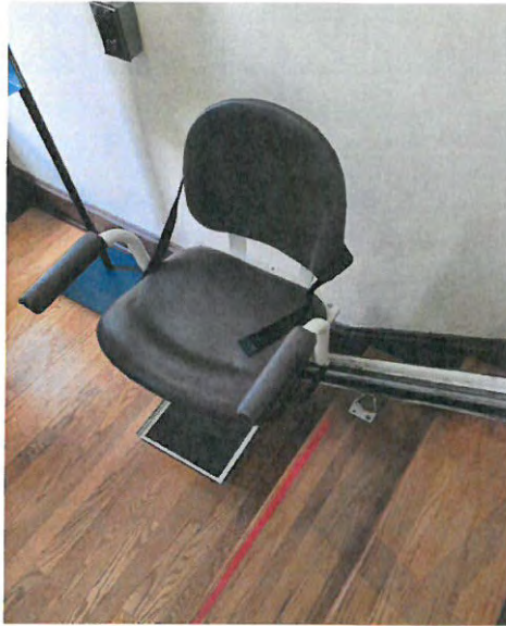
Figure 38: Jamestown Library Accessible Lift
