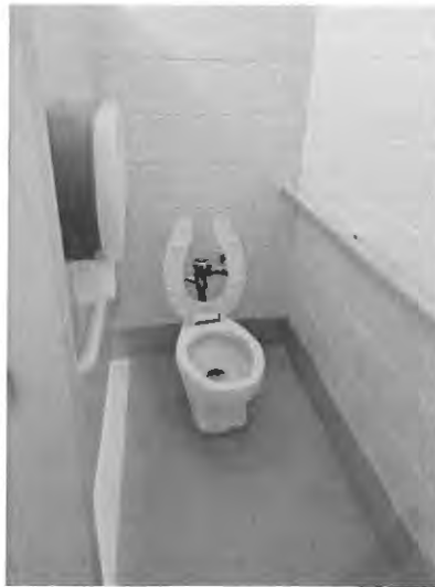
Figure 66: Jamestown Public Park Toilet Room Stall View 3
