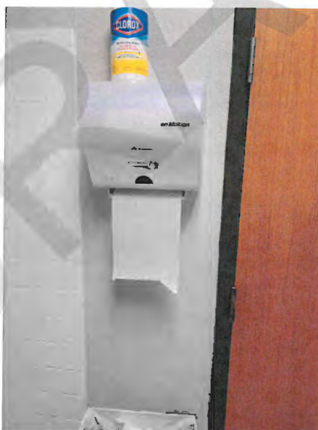
Figure 29: Jamestown Fire Station Men's Towel Dispenser
