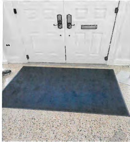
Figure 82: Jamestown Town Hall Entrance Floor
