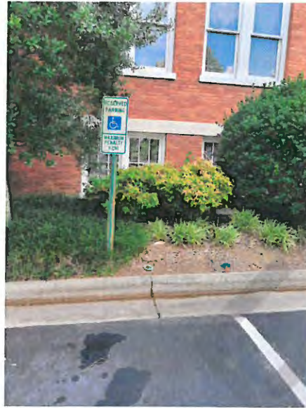
Figure 34: Jamestown Library Accessible Parking Sign
