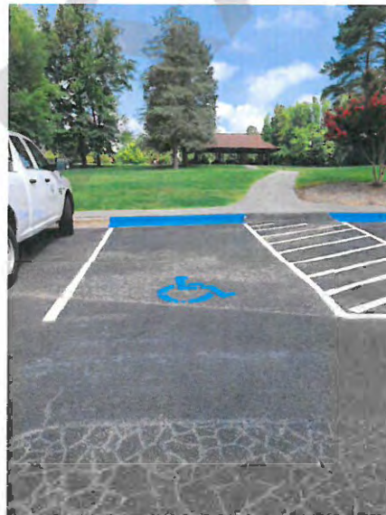
Figure 44: Jamestown Public Park Accessible Parking
