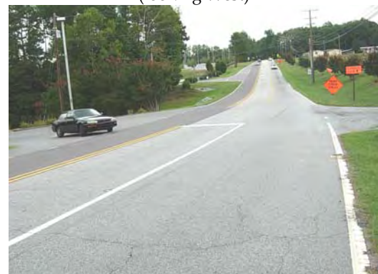
High Point Road West of Intersection at Ragsdale High School (looking East)
