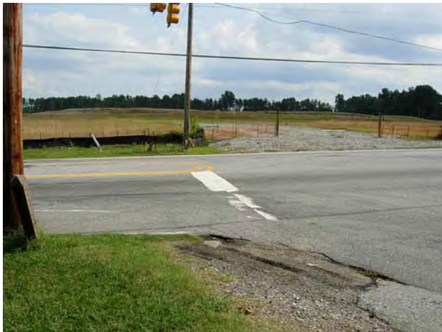
W Main Street at Penny Road (looking South)
