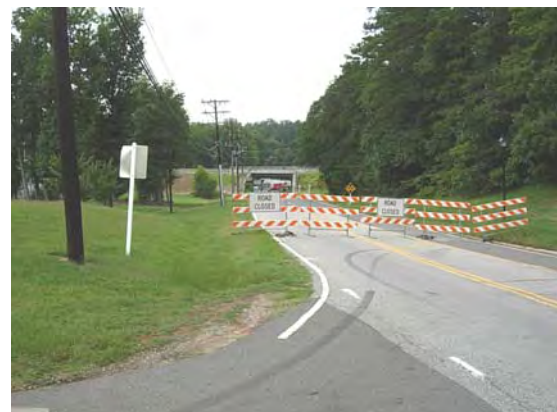
High Point Road (looking Southwest)
