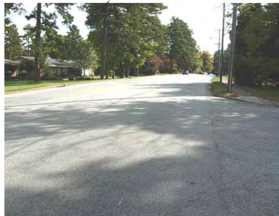
Guilford Road looking south at Forestdale Drive
