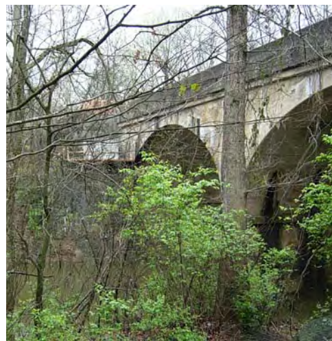
Railroad Bridge over the Deep River
