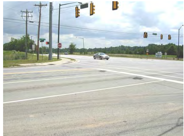
High Point Road Crosswalk (looking South)
