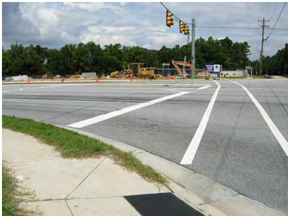
Guilford College Road Crosswalk is 130ft wide (looking East)
