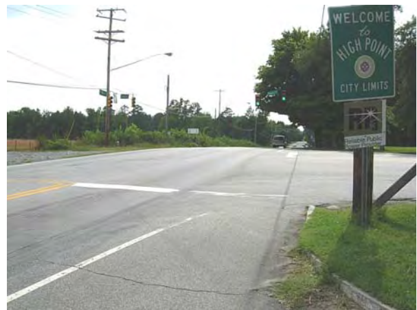
W Main Street at City Limits (looking West)
