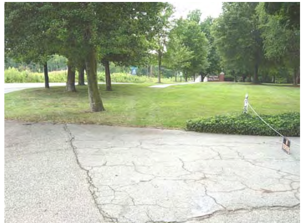
Sidewalk ends along W Main Street (looking West)
