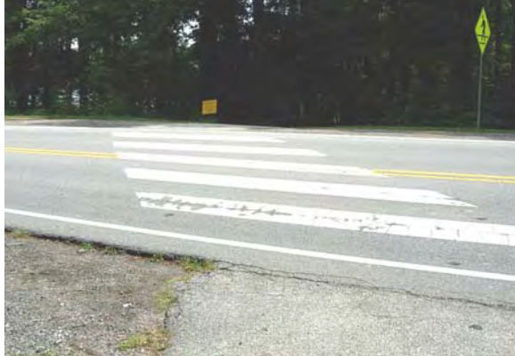
Crosswalk on East Fork Road for Bicentennial Greenway (looking South)
