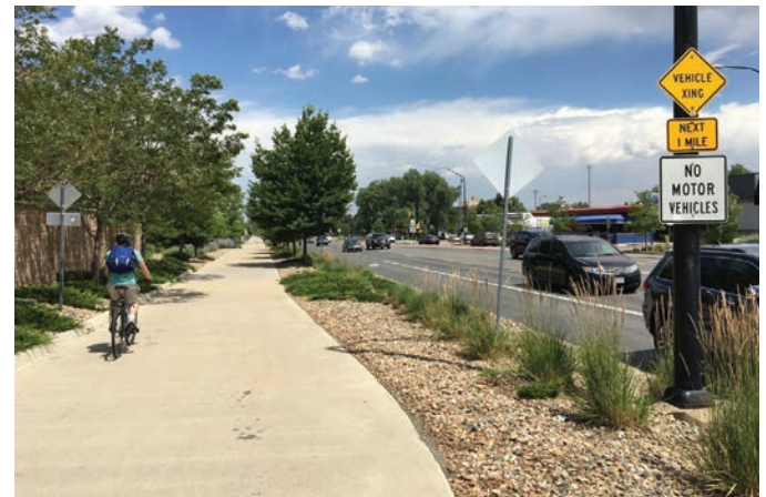
Concrete sidepath with landscape strip
