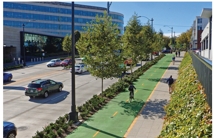
Sidewalk-level two-way separated bike lane
