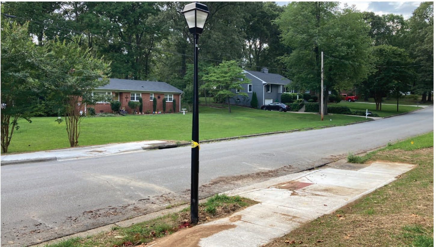
A newly constructed sidewalk on Potter Drive is the latest addition to Jamestown's growing pedestrian network.
