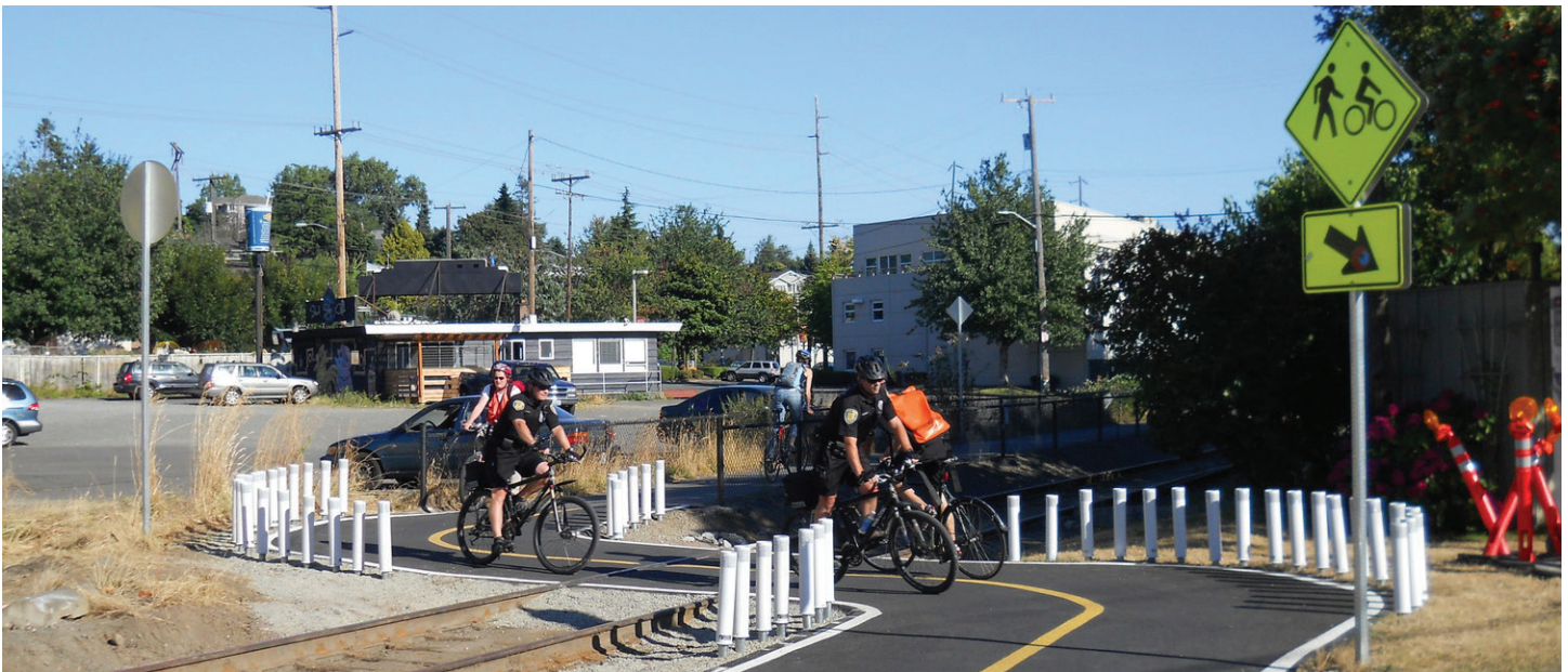
Bike routes that traverse at-grade railroad crossings should cross at a 90 degree angle.
