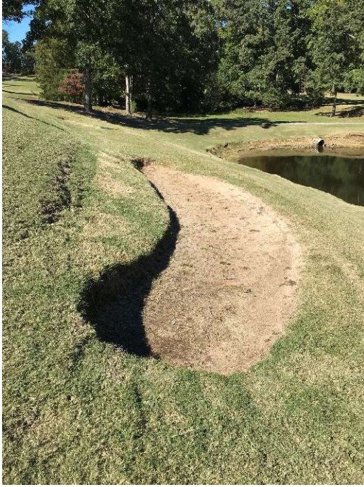
Images of selected sand bunkers at JPGC showing poor conditions with lack of drainage, lack of sand and exposed linings. In addition, there are several small bunkers in awkward locations that are difficult to maintain properly (most notably on par-3 holes # 4 and #17). It is clear that some improvement is needed to this key golf course feature.
