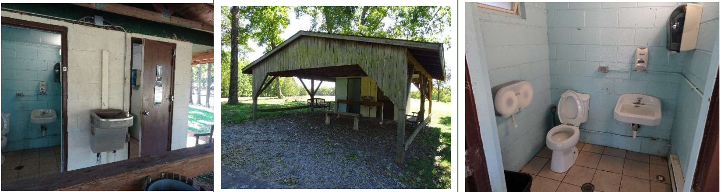
Images of on-course services at JPGC showing extremely poor conditions. Restrooms and drinking stations are being replaced in 2022.
