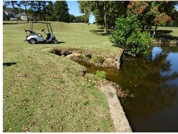
Images of the lake-bank by hole #9 that has been impacted by runoff, which could continue to get worse if not addressed.
