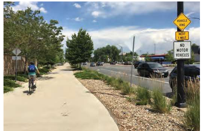
Concrete sidepath with landscape 2 uffer
