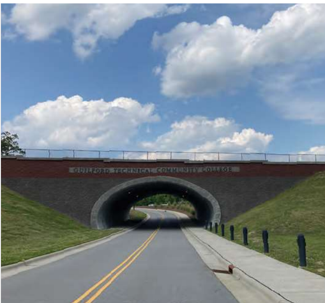
Tunnel under Guilford College Road on GTCC campus
