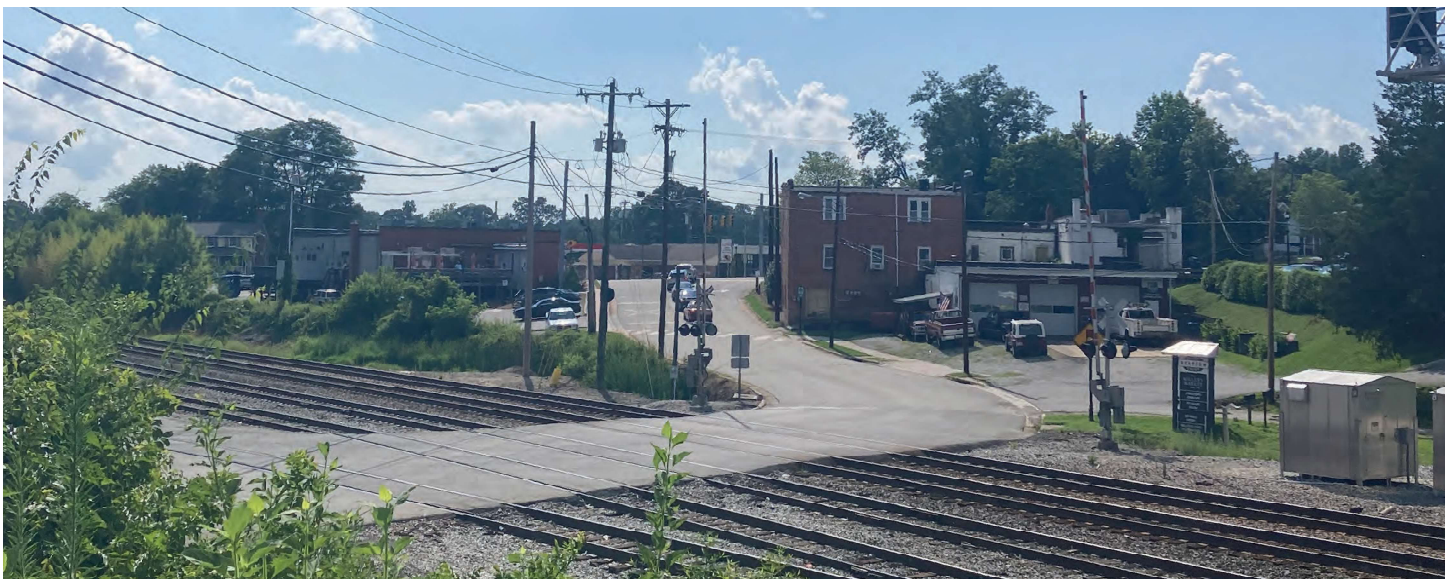
At-grade high speed rail crossing on Oakdale Road
