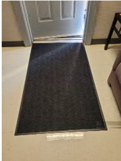
Figure 21: Jamestown Fire Station Entryway Door Mat 1
