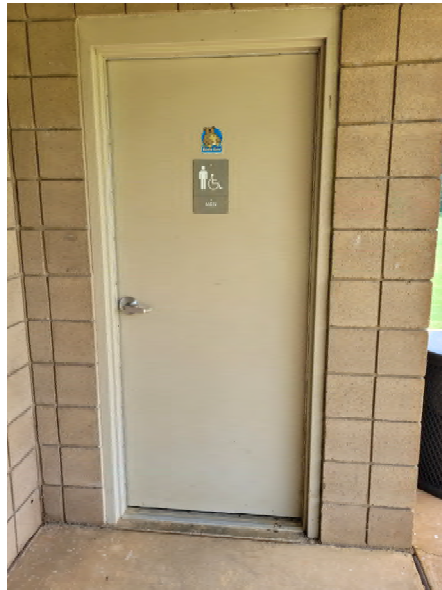
Figure 69: Jamestown Soccer Fields Men's Toilet Room Door
