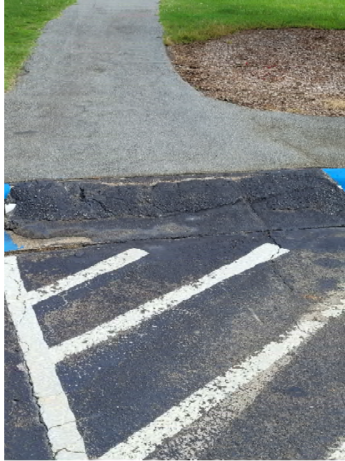
Figure 47: Jamestown Public Park Access Ramp View 2
