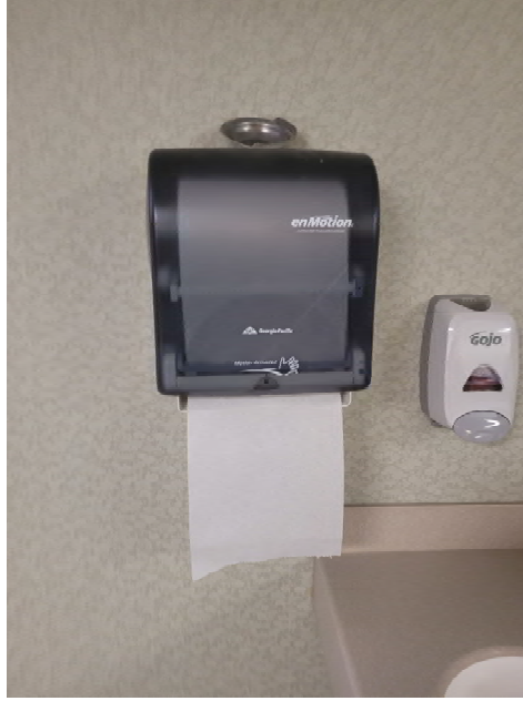
Figure 14: Jamestown Civic Center Toilet Room Towel Dispenser
