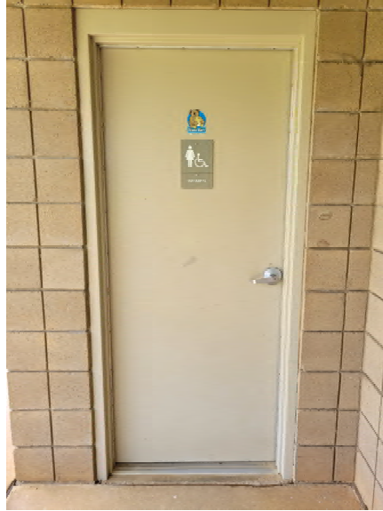
Figure 70: Jamestown Soccer Fields Women's Toilet Room Door
