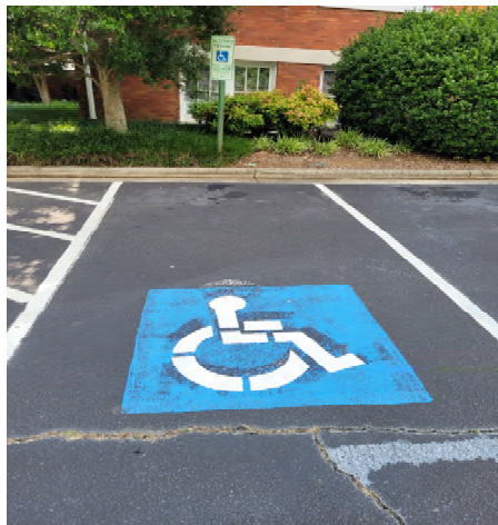
Figure 33: Jamestown Library Accessible Parking
