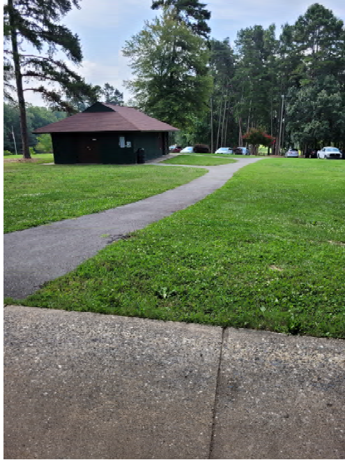
Figure 49: Jamestown Public Park Accessible Route
