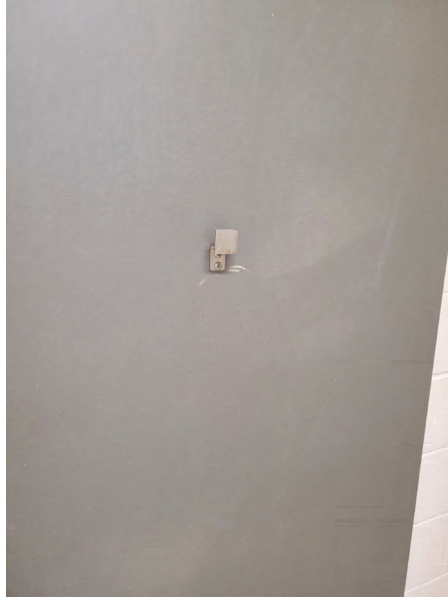
Figure 72: Jamestown Soccer Field Toilet Room Coat Hook View 2
