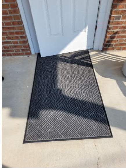
Figure 22: Jamestown Fire Station Entryway Door Mat 2
