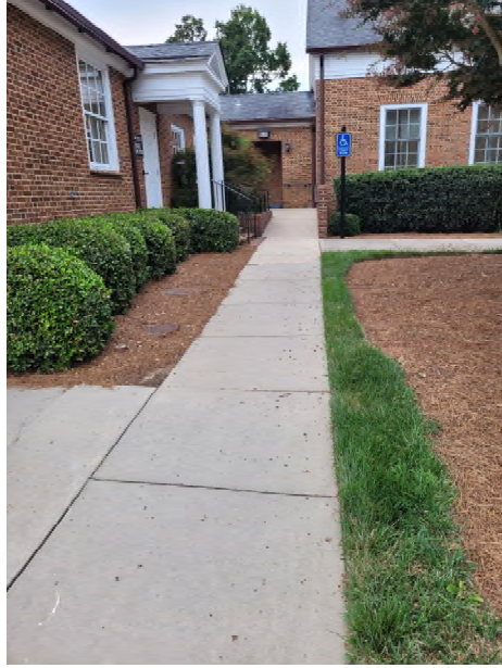
Figure 3: Jamestown Civic Center Entrance Ramp 2
