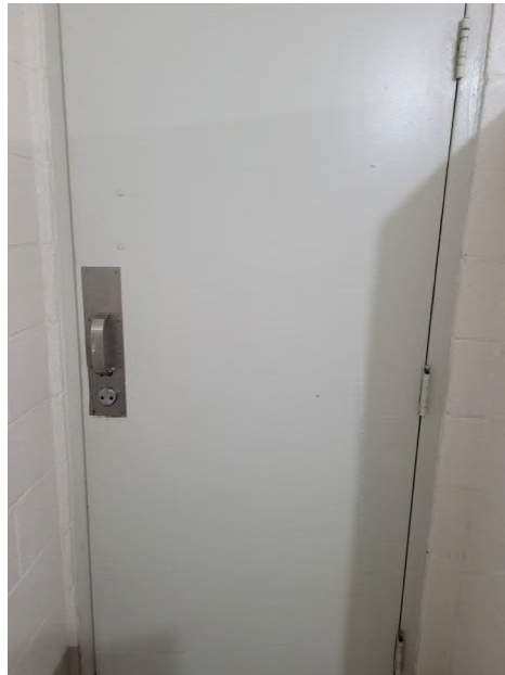
Figure 58: Jamestown Public Park Toilet Room Door View 1
