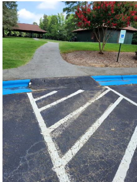
Figure 46: Jamestown Public Park Access Ramp View 1
