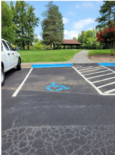
Figure 44: Jamestown Public Park Accessible Parking
