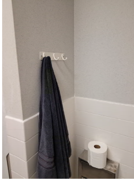
Figure 26: Jamestown Fire Station Women's Toilet Room Coat Hook
