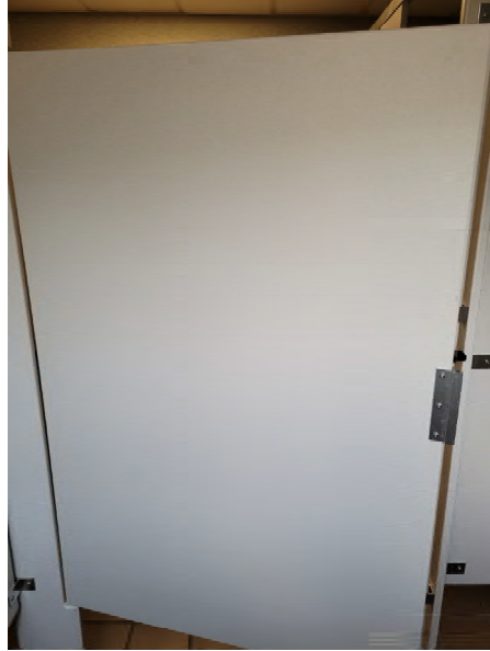
Figure 10: Jamestown Civic Center Women's Toilet Room
