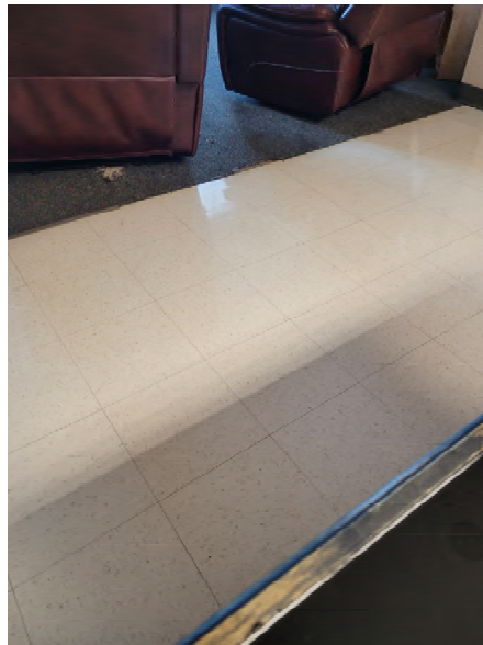
Figure 23: Jamestown Fire Station Walkway
