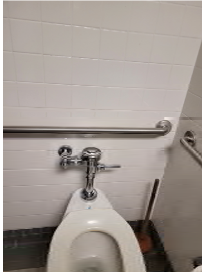
Figure 30: Jamestown Fire Station Toilet Room Grab Bar View 1
