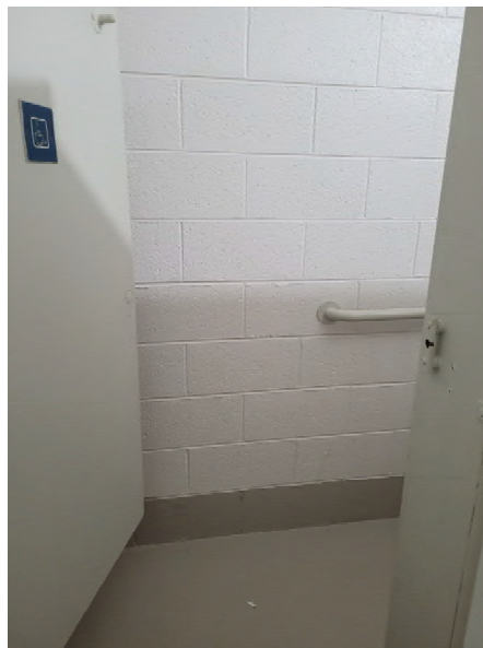
Figure 65: Jamestown Public Park Toilet Room Stall View 2
