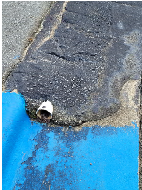
Figure 48: Jamestown Public Park Access Ramp View 3
