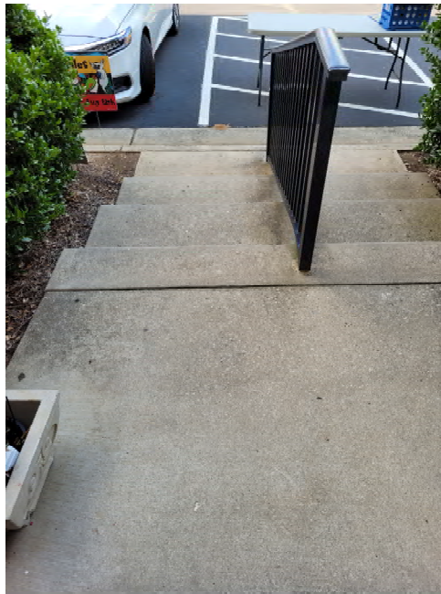
Figure 37: Jamestown Library Front Entrance
