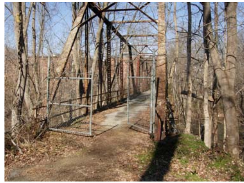
12. Existing bridge below Oakdale Mill dam
