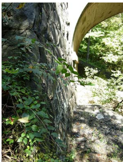
5. Area under NC Railroad bridge looking north
