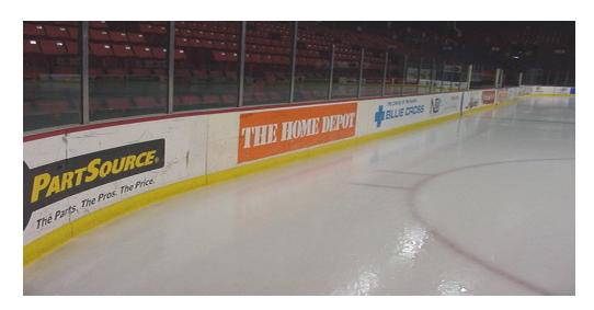
The entire system consists of 68 sections of dashers to accommodate a 200' x 85' ice surface. This dasher system consists of one 16' (2 sections at 8') outside swinging Zamboni gate (located in right corner when standing on ice looking at end). One corner Referees gate, four players box gates and two penalty box gates. There are 66 aluminium glass supports that can accommodate 6'-8' glass or acrylic and there are 62 aluminium supports that can accommodate 4'-6' glass or acrylic.
