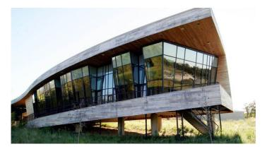
The building can be built at elevation using materials that allow inundation or can be constructed above flood elevation which would allow a variety of specifications. (Dallas, TX)
