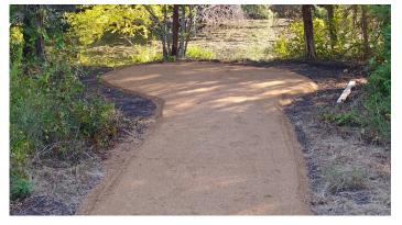
An decomposed granite can provide a more sturdy walking surface and still have low impact during construction.
