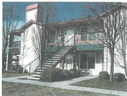
Open, visible entry stair and corridor.
