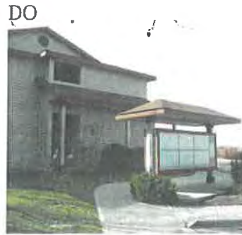
Mailbox consistent with the main structure.
