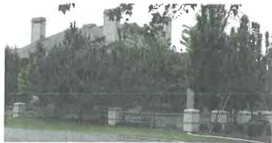
Wrought-iron fence with masonry posts enhanced by landscaping along the property line.
