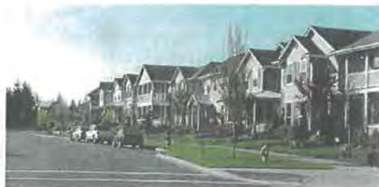
Consistency in the roofline and bulding form.
