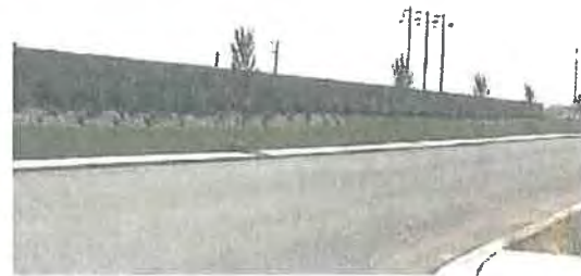
Common RV storage area screened behind the wall.
