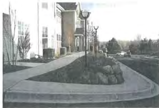
Safe pedestrian access along with vehicular access.
