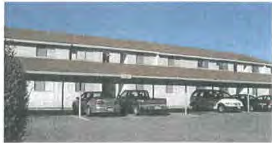
Long, continuous carport in the front.
