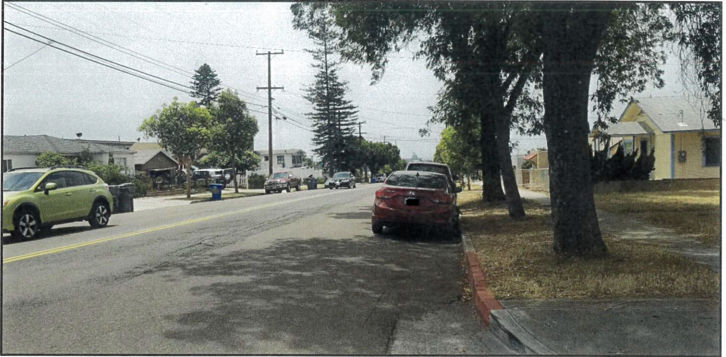
Location of proposed safety enhancements on the north side of E. 16 th St, west of “K” Avenue (looking west)
