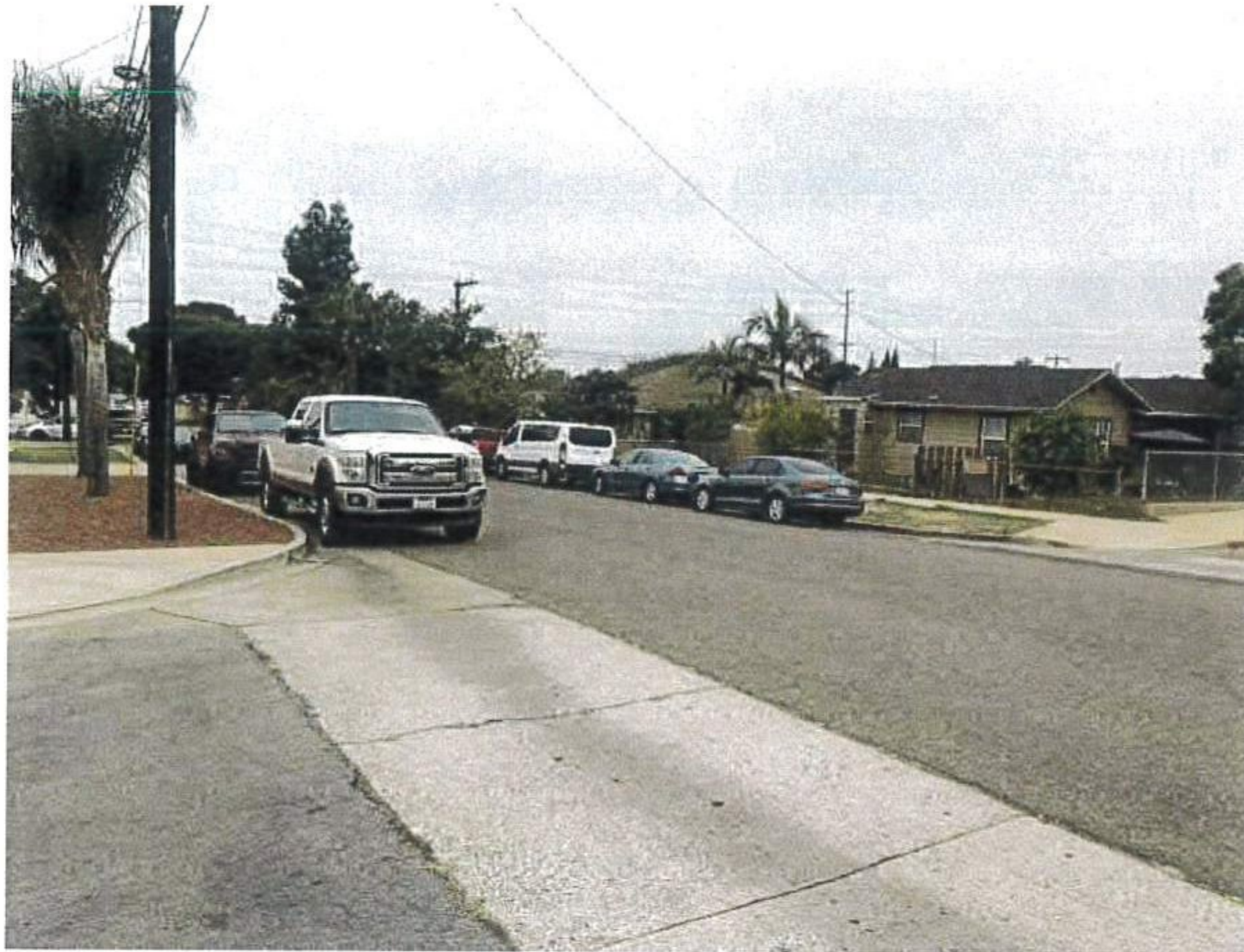
From E Avenue –Northbound looking left (west)
