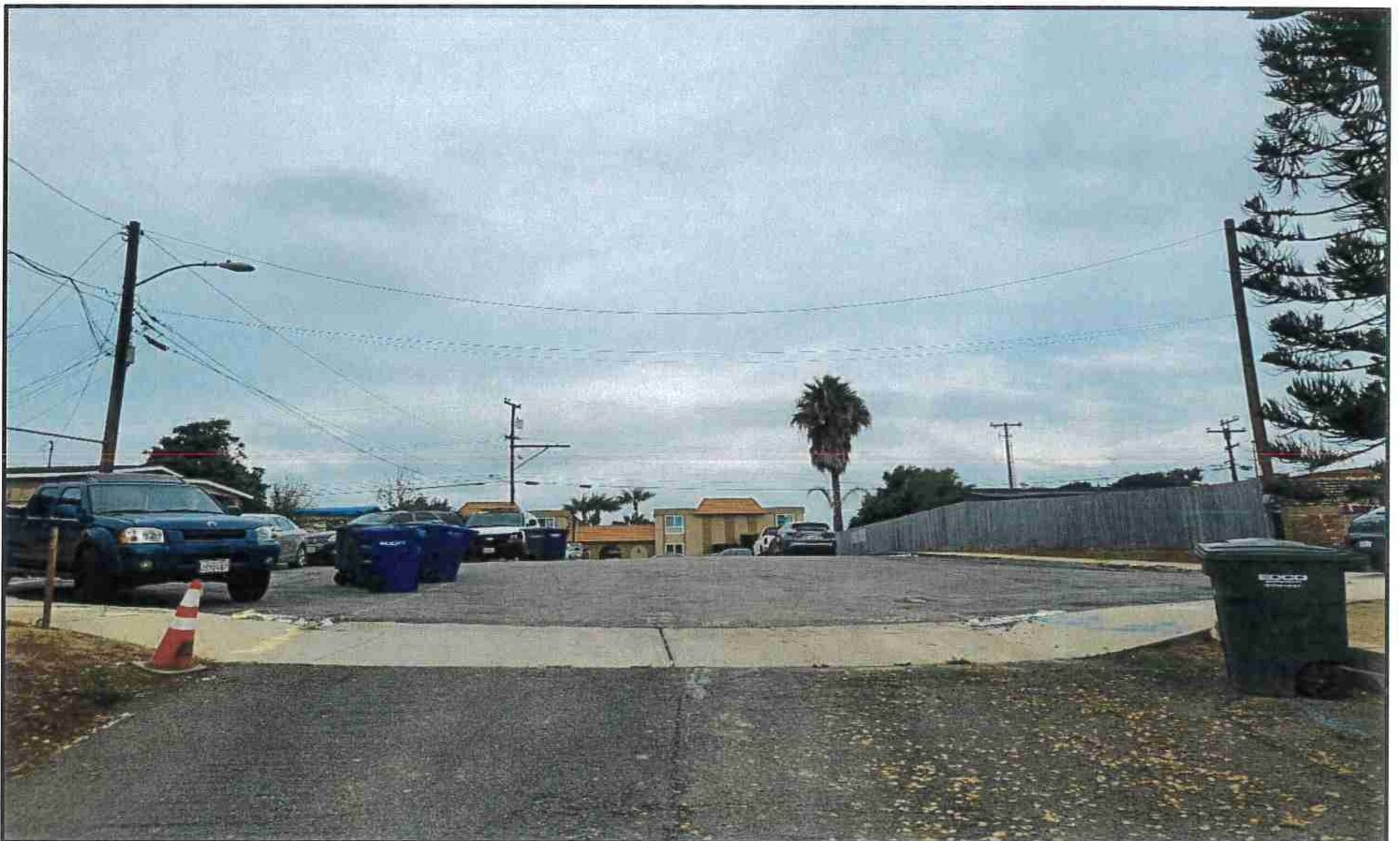
Proposed Residential Parking Permit District "N" – "C" Avenue (looking north)
