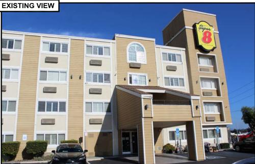
(P) DISH Wireless L.L.C. ANTENNAS AND—RADIOS CONCEALED WITHIN (E) CUPOLA/ENCLOSURE. (E) SHIPLAP SIDING TO BE MODIFIED AND REPLACED WITH FRP MATERIAL. (P) FRP PANEL TO BE PAINTED AND TEXTURED TO MATCH BUILDING.
