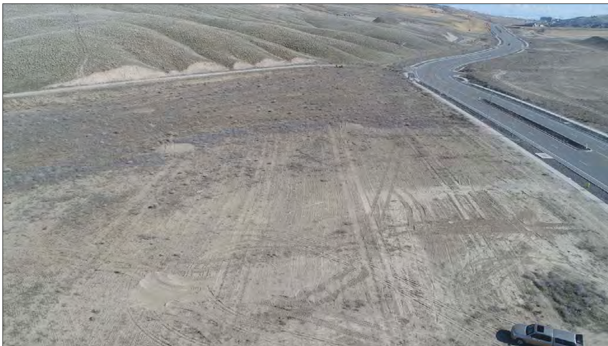
Figure 7. Overview of the Project Area. View to the east.
