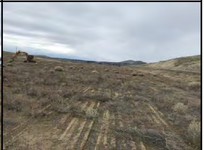
View of site conditions looking NW from TP-14
