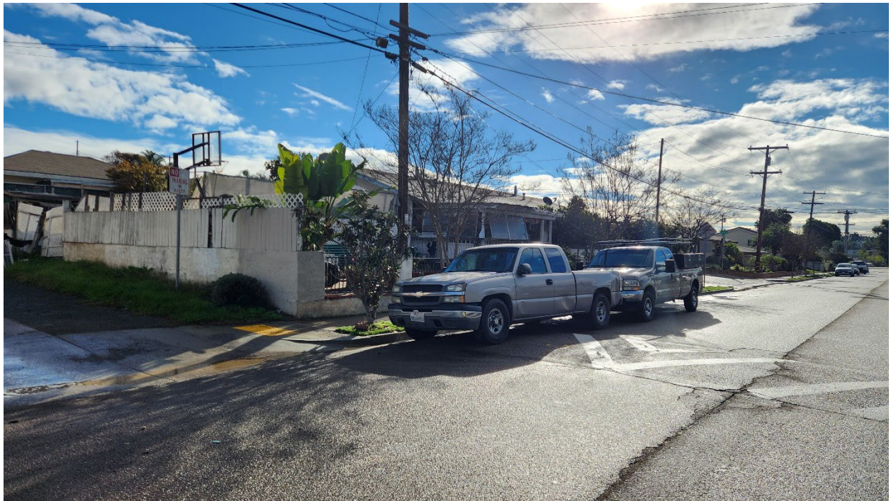
Location of proposed red curb “No Parking” on “M” Avenue (looking east)
