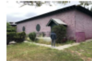
Current Accessible Entry
