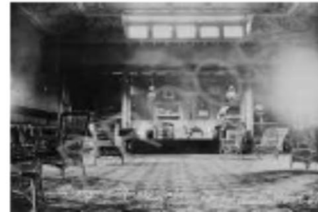
Interior Looking towards Mezzanine
