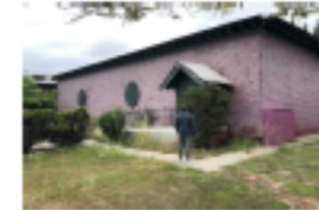
Current Accessible Entry
