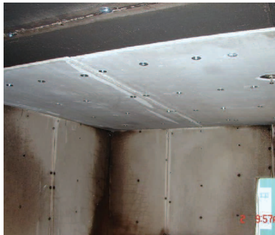
Figure C-5: Additional construction of burn room walls and ceiling and deluge sprinkler head.
