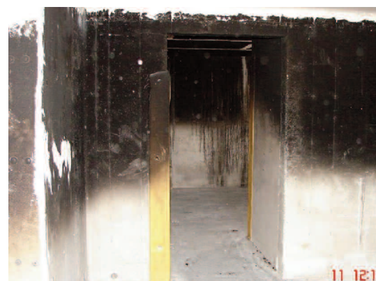
Figure C-7: Interior View of Burn Prop
