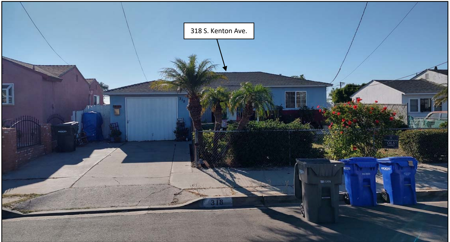
Photo of the driveway and garage at 318 S. Kenton Avenue (Looking South-West)
