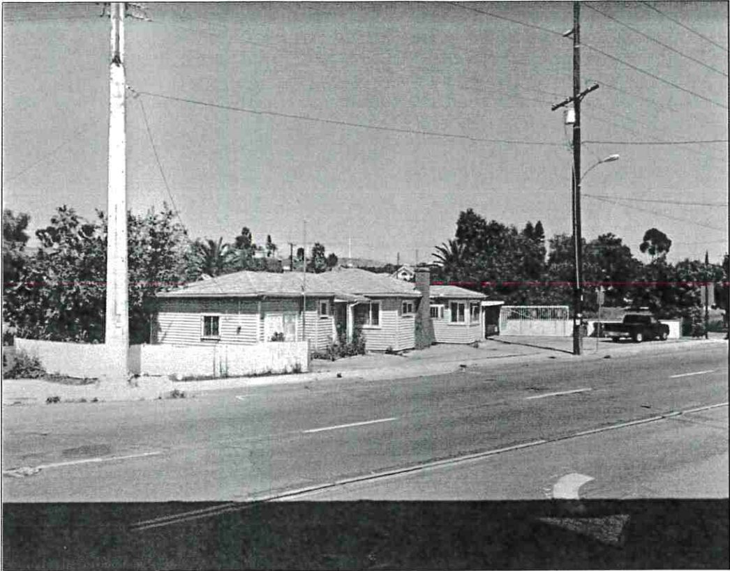
Existing residence looking northeast from Sweetwater Road
