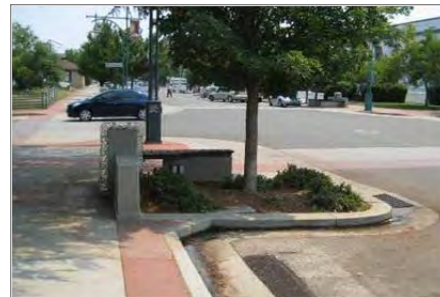
Curb extensions can be a good location for pedestrian amenities, including street trees.
