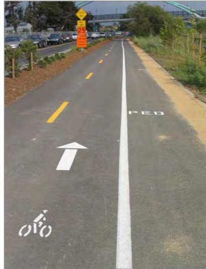
Centerline striping and directional arrows encourage bicyclists to provide space for other trail users to pass.
