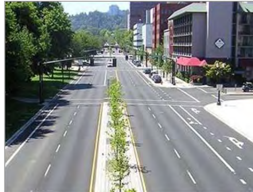
This street in Portland, Oregon previously had 13' lanes which were narrowed to accommodate bicycle lanes without removing travel lanes.
