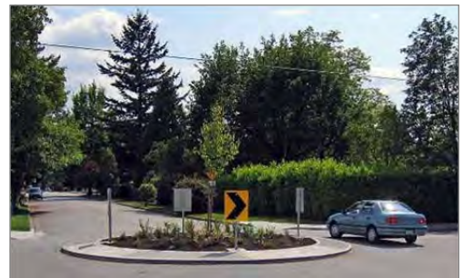
Traffic circles provide an opportunity for landscaping, but visibility should be maintained.
