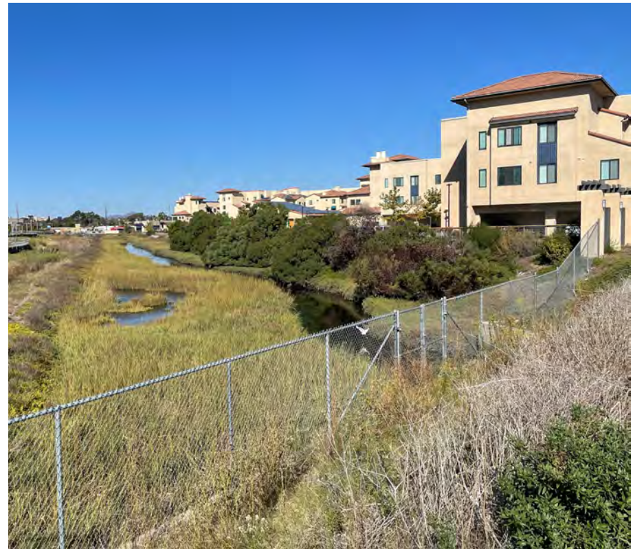
Multi-family residential development adjacent to Paradise Creek
