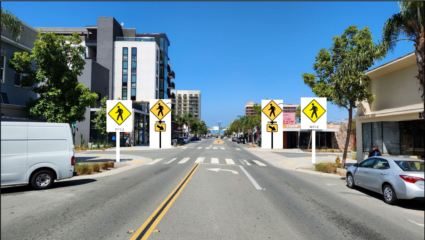
Location of proposed RRFB and warning sign for westbound traffic at 8 th Street and A Ave (looking west)
