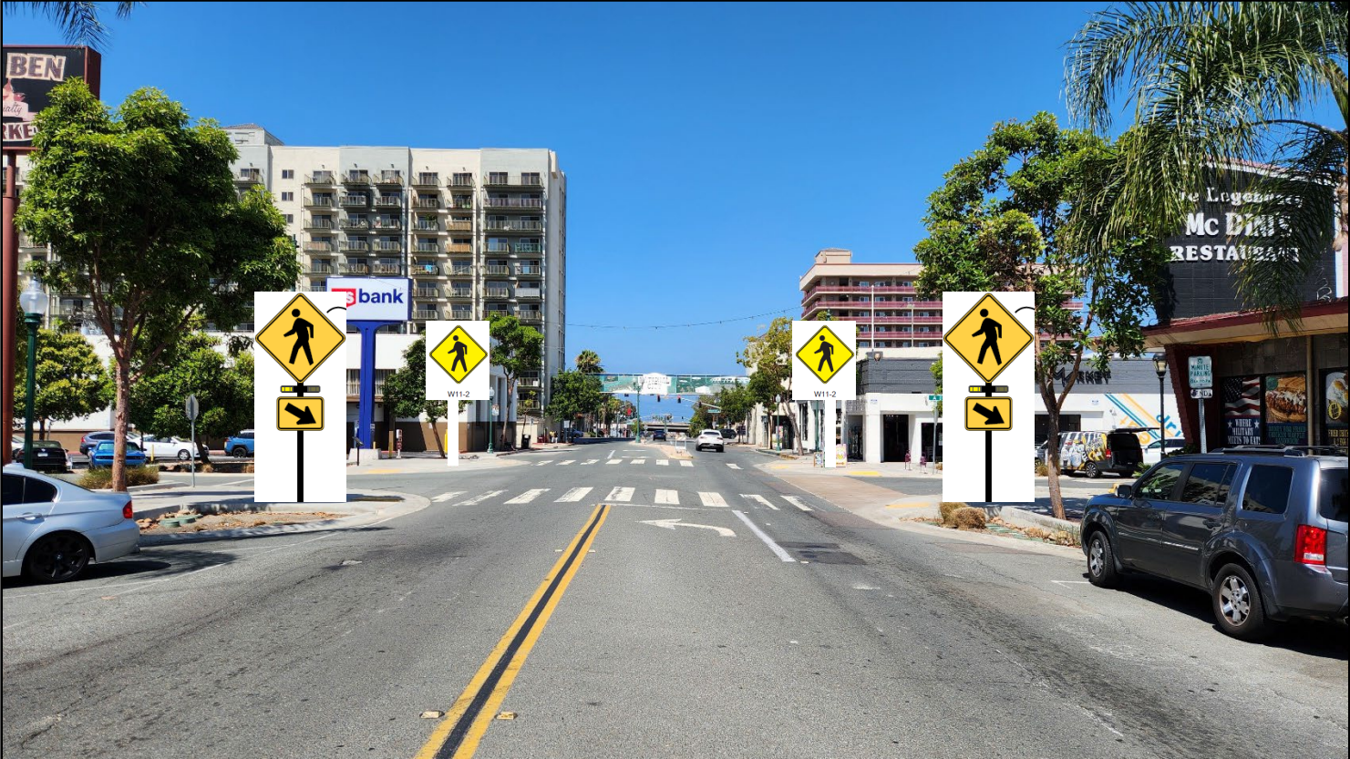
Location of proposed RRFB and warning sign for westbound traffic at 8 th Street and A Ave (looking west)
