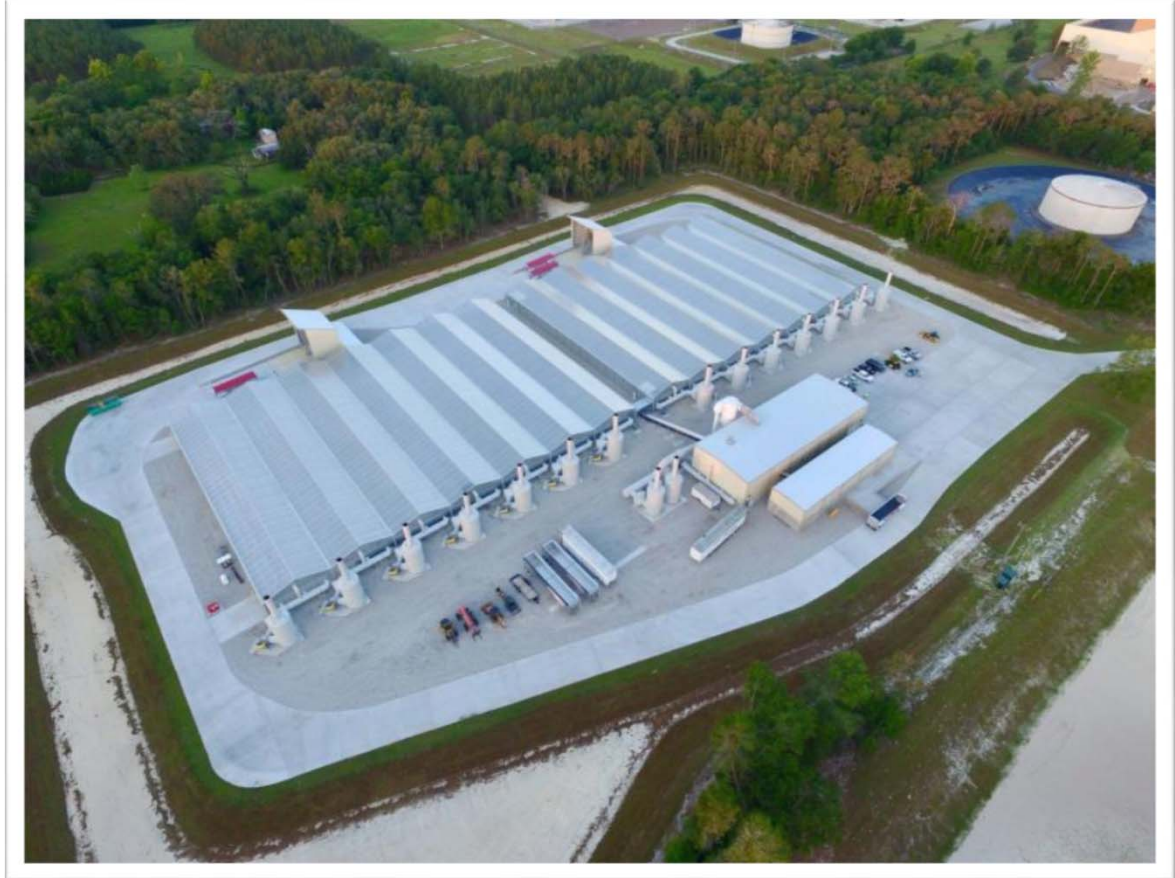
Merrell Brother Biosolids Plant, Pasco County, FL
