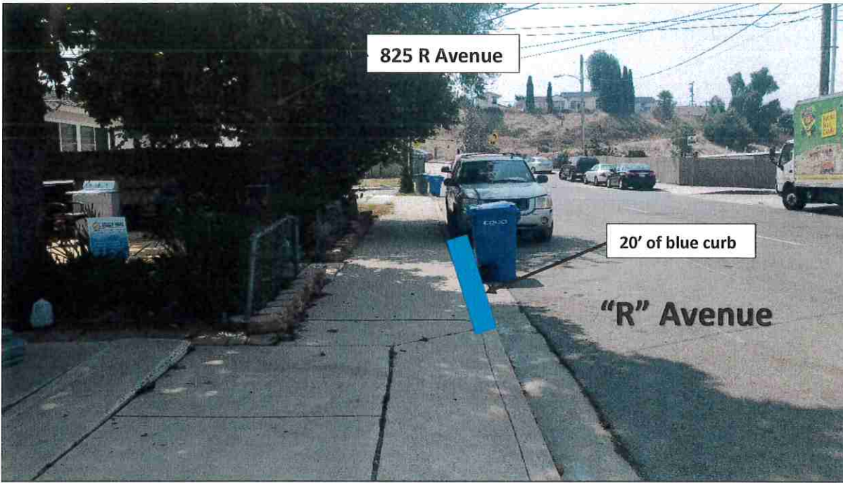
Location of proposed blue curb disabled persons parking space in front of 825 R Avenue (looking south)
