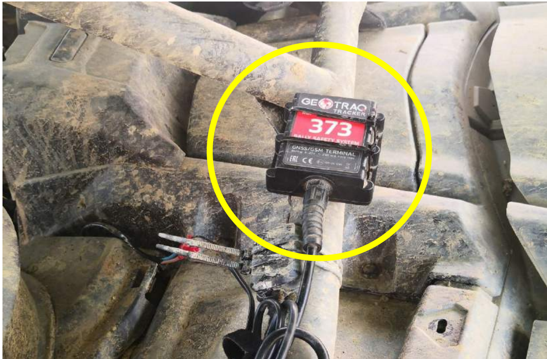
Installation of the GPS TRACKER on the railing of ATV using cable ties.
