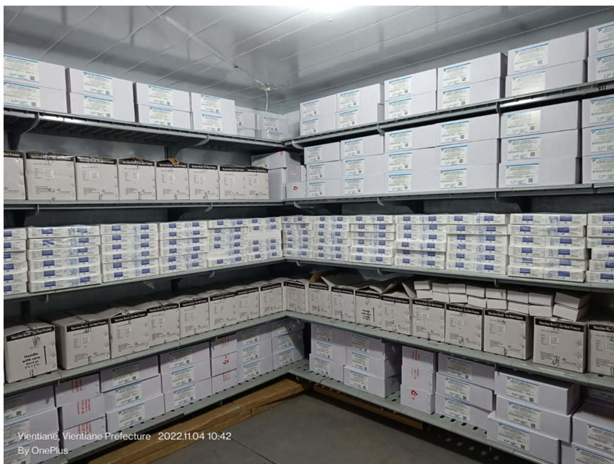
Figure 17: Well-maintained walk-in cold room at central vaccine store, NIP
