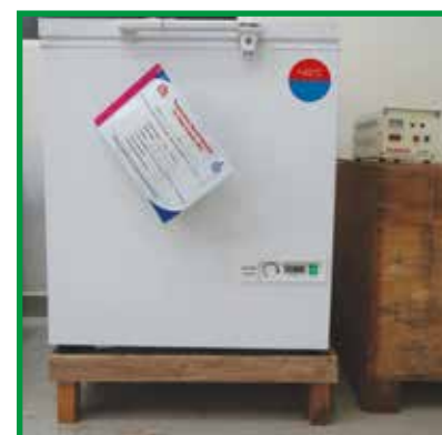
Deep Freezer placed on wooden stand with independent stabilizer and temperature log book
