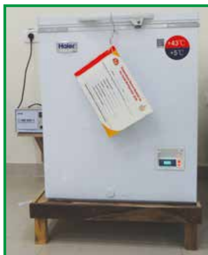
ILR placed on wooden stand with independent stabilizer and temperature log book
