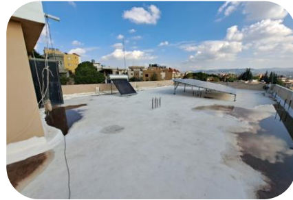
Roof photos from different perspectives
