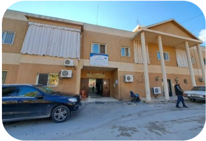
Building photos from different perspectives
