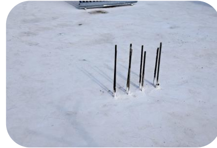
Roof construction type
