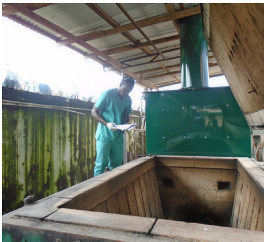
FIG. A4 – Inspecting an incinerator in Liberia
