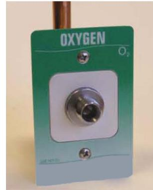
which is serviceable without shutting off the gas service and is capable of supporting 10 pounds @ 2" from the nameplate without leaking.
