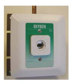
of an inch (1.3 cm to 3 cm). The name of the gas service shall be permanently marked on the outlet bracket and the outlet. The outlet's rough-in supply tube shall be a 7 inch (18 cm) length of 1/2 O.D. copper Type K for all gas services and labeled with the name of the gas service.
