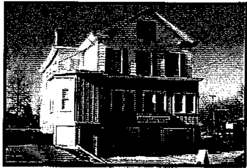
Ø This front addition disregards the scale, massing, details and materials of the main building.
