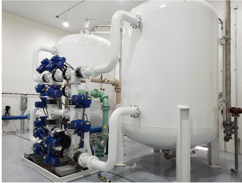
GAC treatment system constructed in Warrington Township for the North Wales Water Authority.
