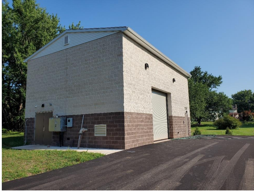
GAC treatment building constructed in Warrington Township for the North Wales Water Authority.
