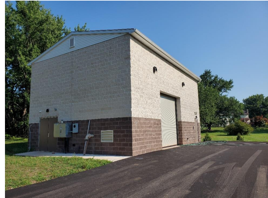
GAC treatment building constructed in Warrington Township for the North Wales Water Authority
