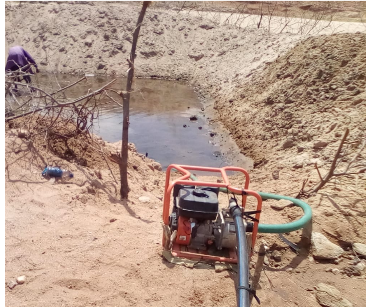
Image: A diesel-powered pump pumping water from a shallow pool of water.
