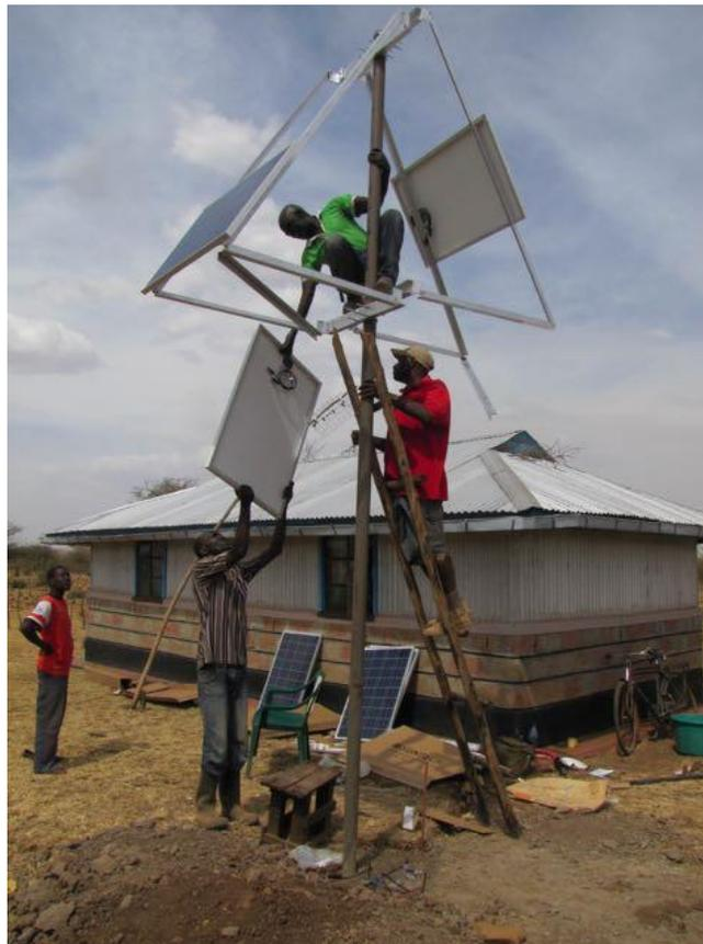
Photo 1 Elaborate and expensive pole mounting for PV SMART systems
