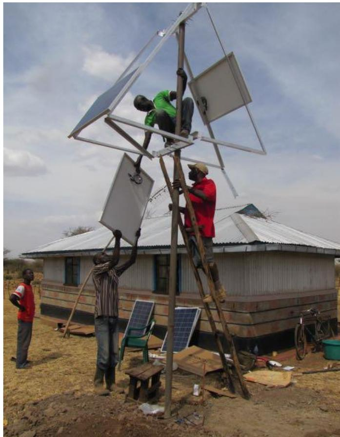
Photo 1. Installing pole mount solar arrays for PV SMART project in Kenya
