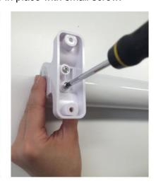
3. Hold the heater against the wall and mark the position of the fixing holes. If fixing to a studded wall, or a Wooden surface, use the large screw and wall plug. If the wall is hollow, or you are drilling into masonry, using the pilot holes as guide, drill again using a 6.5mm drill bit and insert a wall plug into each hole. Once holes are prepared, mount the tube and secure.
