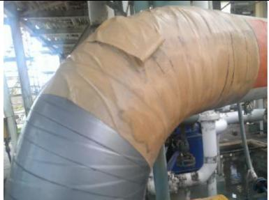
Remark: The surface's Anti-Corrosion Materials did not recovery by Furuto's SOP during one year (2013) checked. (it's just only use a packaging tape for temporary repaired, which couldn't Anti-UV, Water Tight & Air Tight). Tip: Enlarge the PDF file to see the photo in details.
