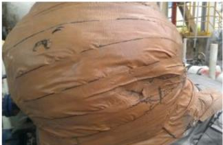
Remark: The surface's Anti-Corrosion Materials did not recovery by Furuto's SOP during one year (2013) checked. (it's just only use a packaging tape for temporary repaired, which couldn't Anti-UV, Water Tight & Air Tight).
